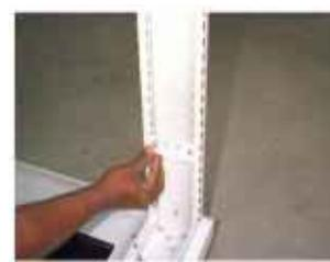
7. Install the panel mounting brackets within the picture frame. For 19" offset mounting 3+3 of these brackets must be installed along one side of the cabinet while 6+6 must be installed on the opposite side where the offset is required. Insert the retainer clips as shown
