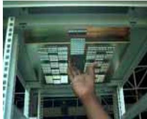
17. The Fan Housing Unit is installed to the underside of the top cover by utilizing the four studs provided.
