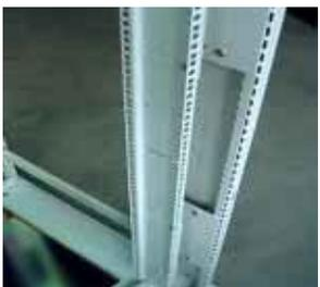
15. The 19" equipment mounting angles are fastened to the 'U' channel brackets on the offset side. On the opposite side of the cabinet the 19" angles are to be fastened directly to the panel mounting brackets.
