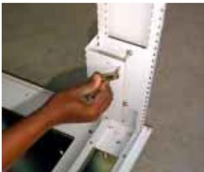
13. Install the offset brackets. Three of these will be needed at the front and three at the back along side of the cabinet where the offset mounting is required. Each of these offset brackets are to be fastened to a pair of the panel mounting brackets installed earlier.
