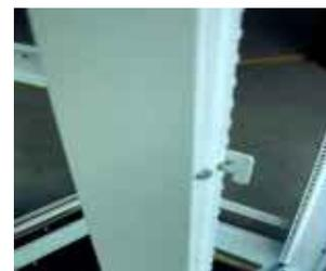
9. On the lock side of the door three "Bump-On" buttons should be positioned, one at the centre as shown and the other two at the top and bottom corners of the door.
