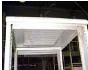
6. Fasten the top cover assembly to the two "Picture Frames" in the same way as the bottom cover
